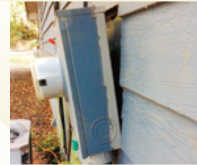
HB Next technicians are alerting customer-owners to hazards like meter bases that need attention.
